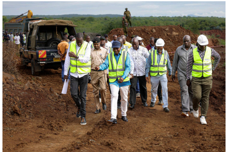
H.E. Deputy President Prof. Kithure Kindiki inspected the ongoing construction of the Mogotio–Lake Bogoria–Kisanana–Kamukunji Road in Mogotio Constituency, Baringo County, on 17th April 2026.
