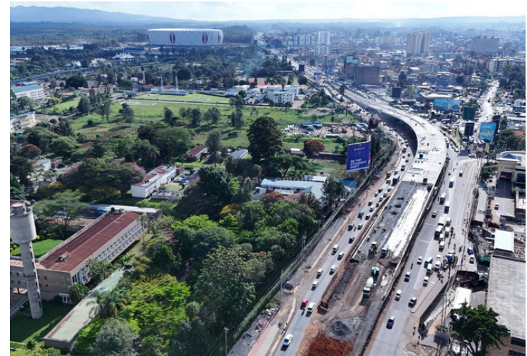
Construction of the Ngong Road–Naivasha Road overpass is nearing completion.
