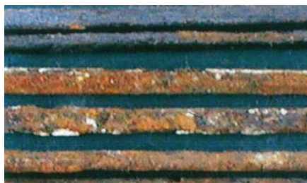
Steel corrosion rate survey
