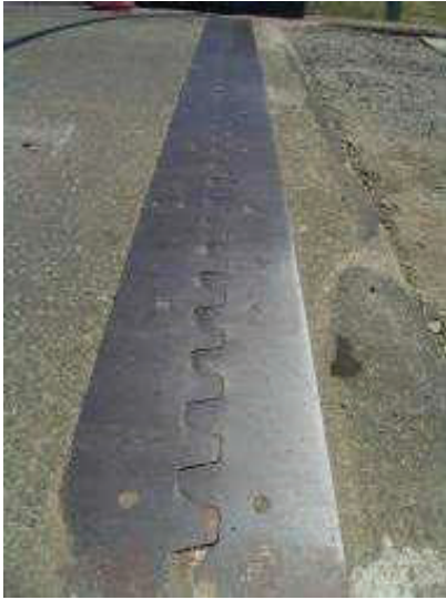
Abnormal clearance of expansion joint
