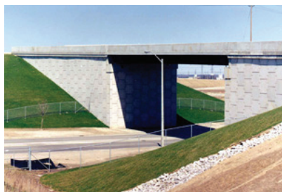
1. Full-retaining ( h > 5\text{m} )
