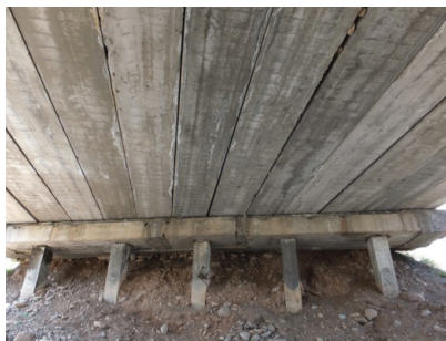
3. Spill through (open)
