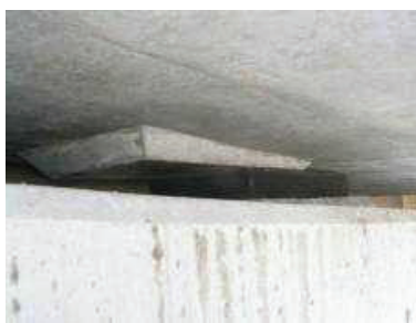
Displacement of rubber bearing
