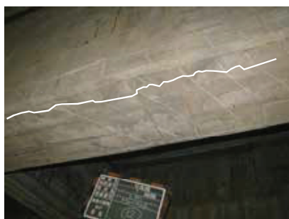
Crack/spalling (T-girder)
