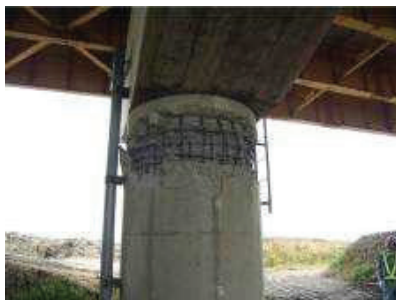
Flaking of covered concrete (Parallel part)
