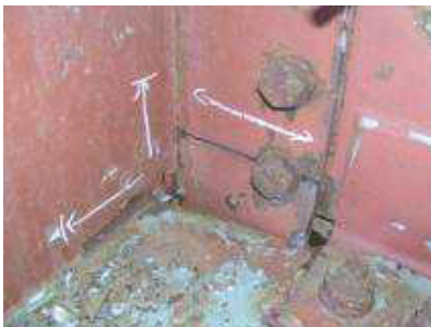
Cracking of vertical stiffener and gusset
