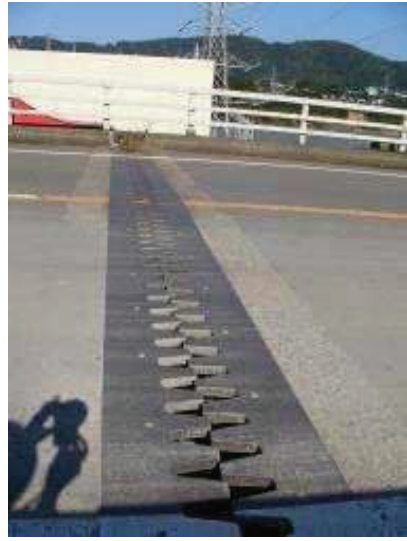
Abnormal clearance of expansion joint
