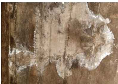
Efflorescence
