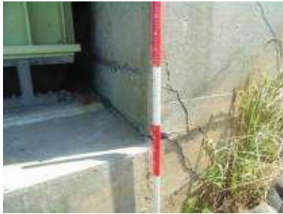
Cracking of parapet base
