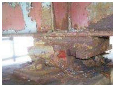
Side block rupture
