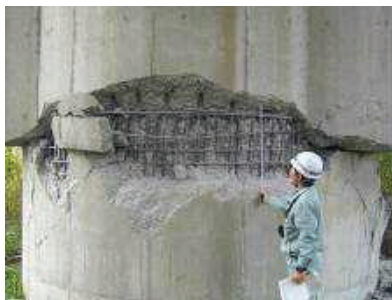
Flaking of covered concrete (Parallel part)
