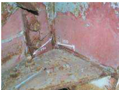
Cracking of vertical stiffener and gusset
