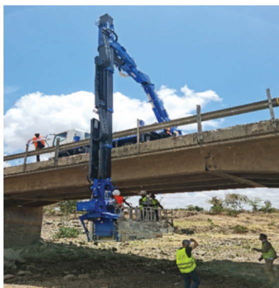
Inspection using a bridge inspection vehicle
