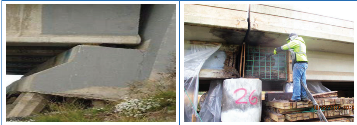
Figure 3.81 Sample photos of gap error of girder end
