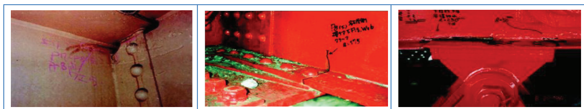
Figure 3.35 Sample photos of cracks of steel members
