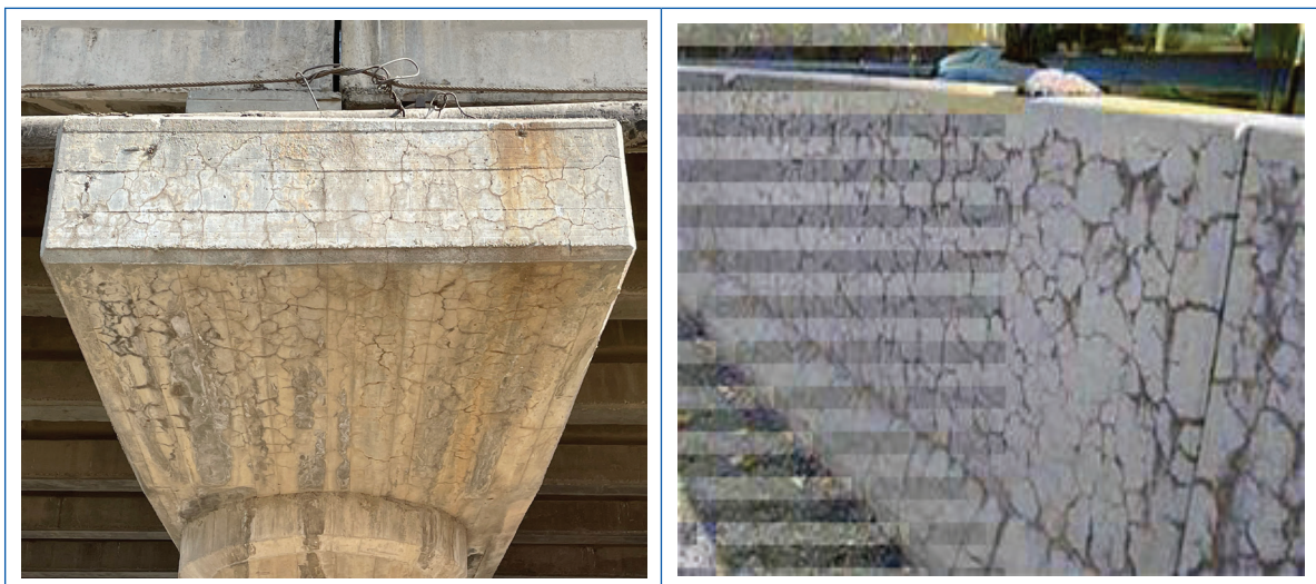
Figure 3.14 Sample photos of ASR
