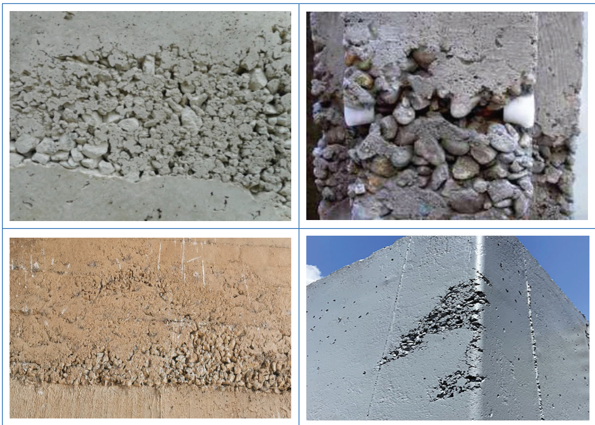
Figure 3.10 Sample photos of honeycomb
