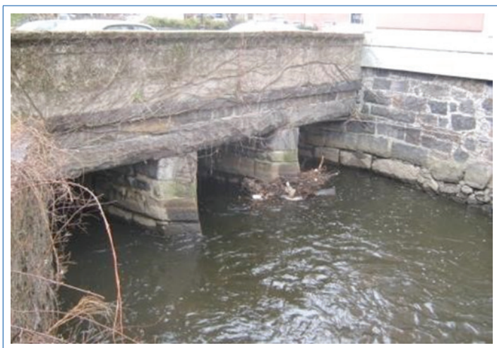
Figure 2.31 Granite slab bridge
