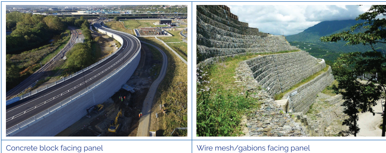
Figure 3.61 Sample photos of reinforced earth retaining structures
