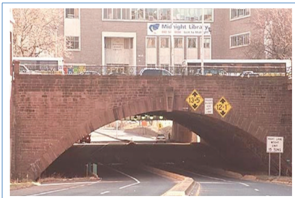
Figure 2.33 Brick arch and spandrel walls
