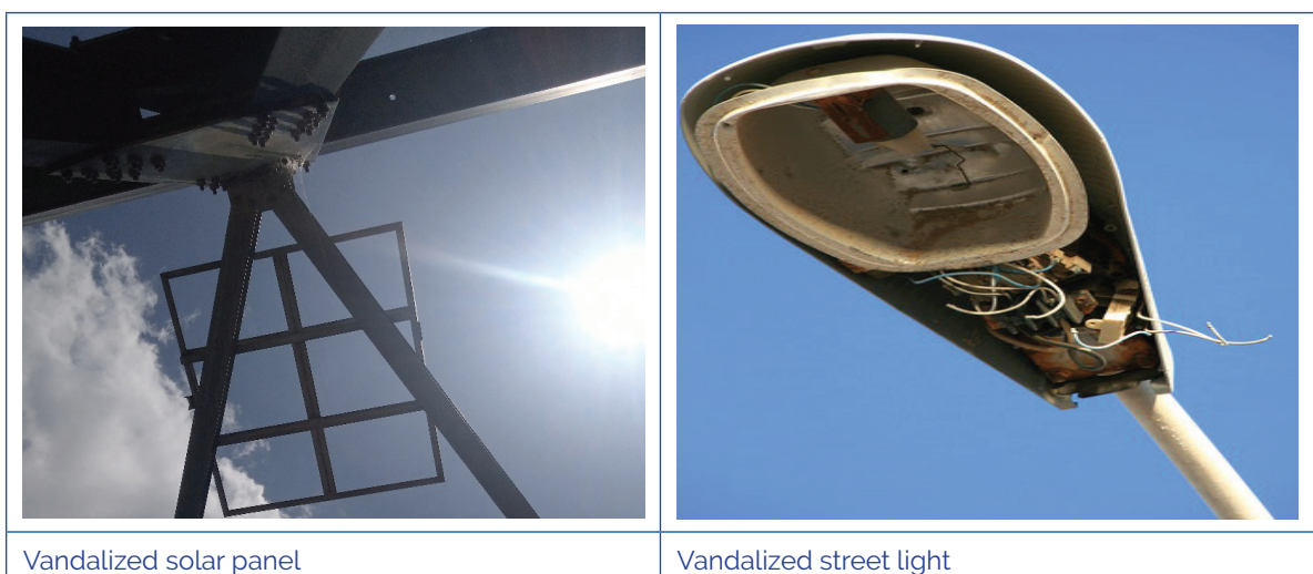
Figure 3.63 Sample photos of signage deteriorations
