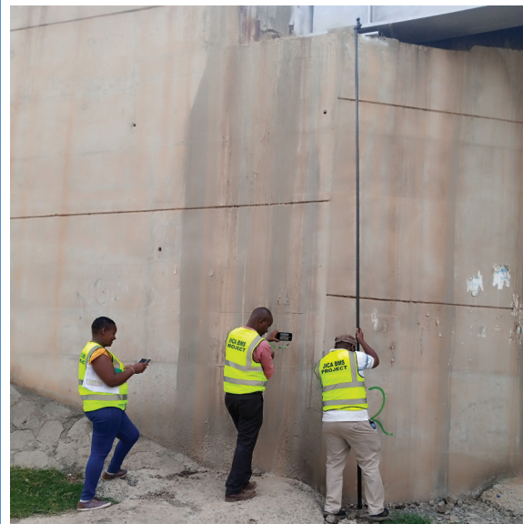
Inspection using a pole camera
