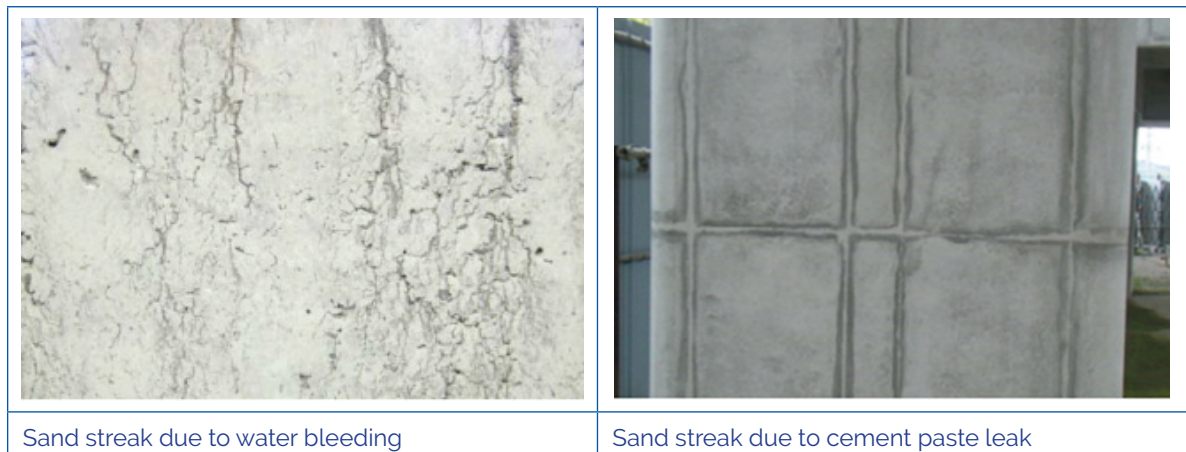
Figure 3.25 Sample photos of sand streak
