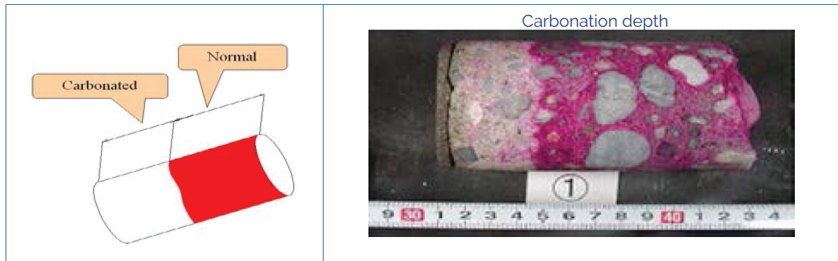
Figure 7.52 Measurement of carbonation depth on concrete core sample
