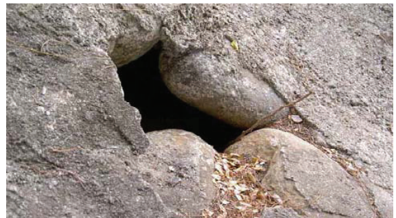
Figure 3.12 Partial replacement of masonry slope protection
