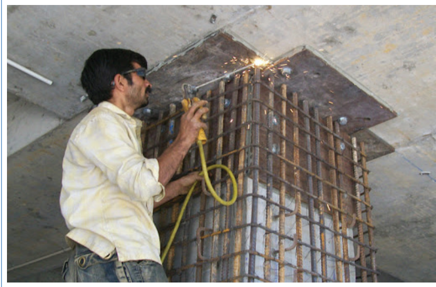
Figure 3.85 Welding of reinforcement bars
