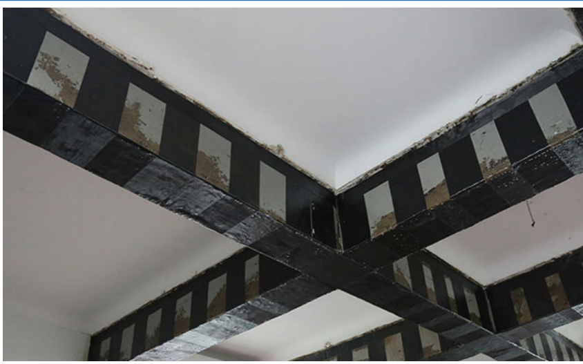
Figure 3.88 Fibre reinforced polymer jacketing
