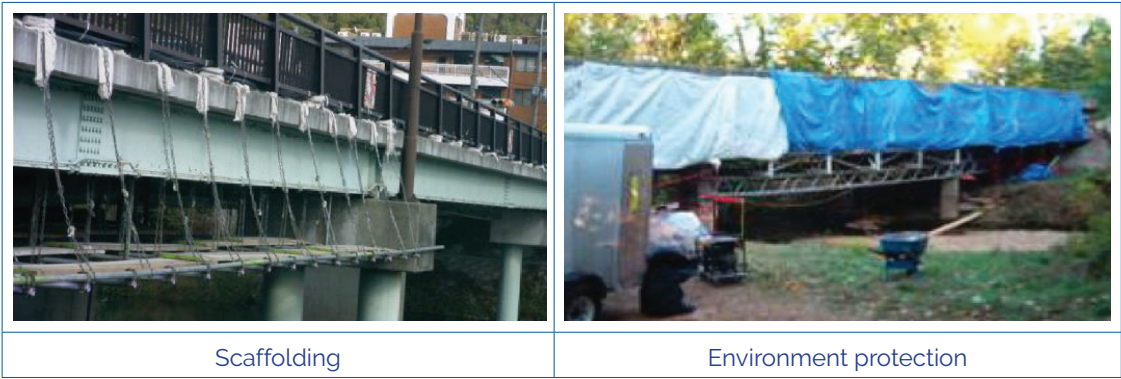
Figure 3.37 Scaffolding for safe repair works and environmental protection
