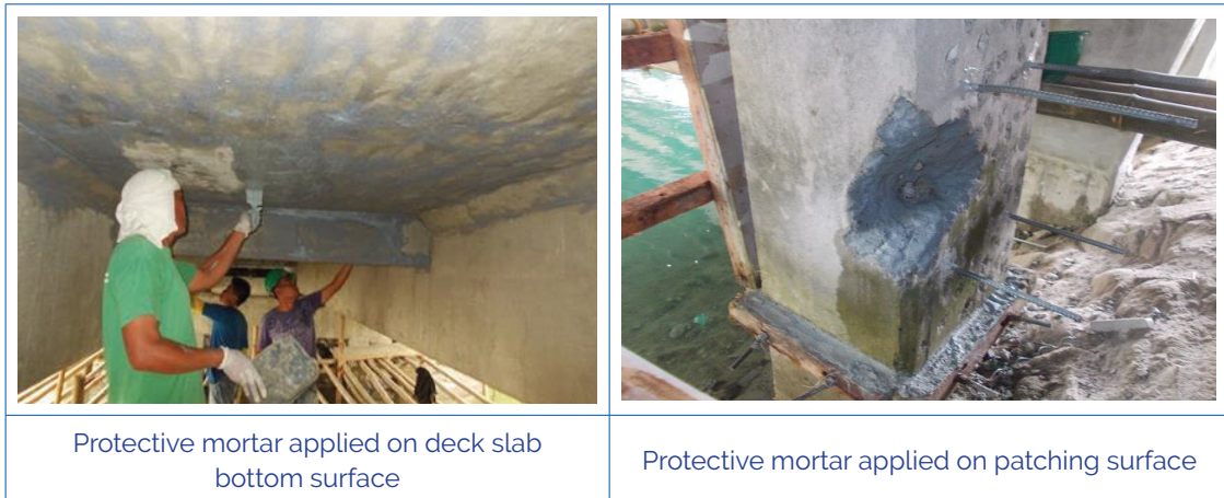
Figure 3.29 Protective mortar applied on deck slab bottom surface
