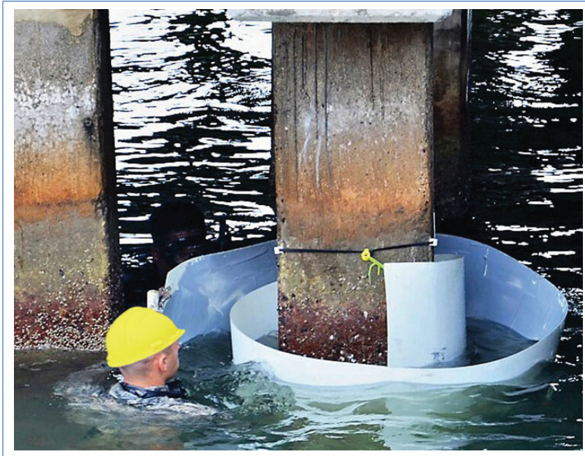
Figure 3.89 Glass fibre reinforced polymer jacketing
