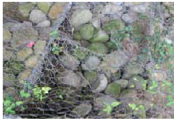
Figure 3.13 Partial replacement of gabion wire mesh and stone
