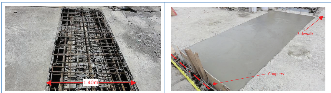
Figure 3.28 Fast setting concrete for continued deck slab
