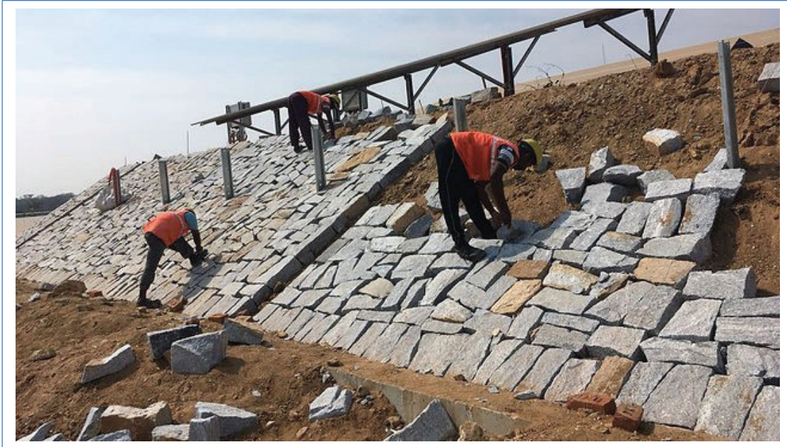
Figure 3.92 Laying of stone pitching
