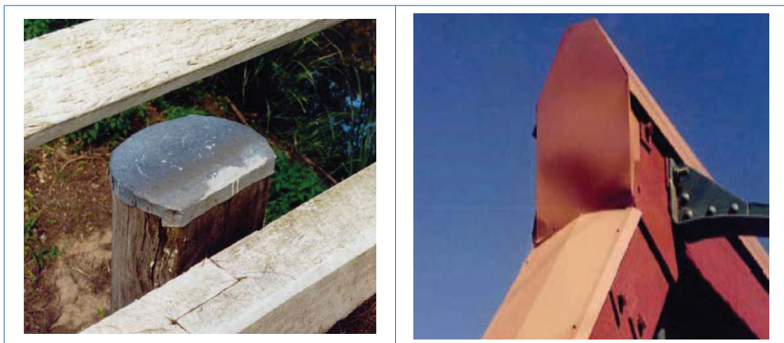
Figure 3.58 Photo of installed flashings
