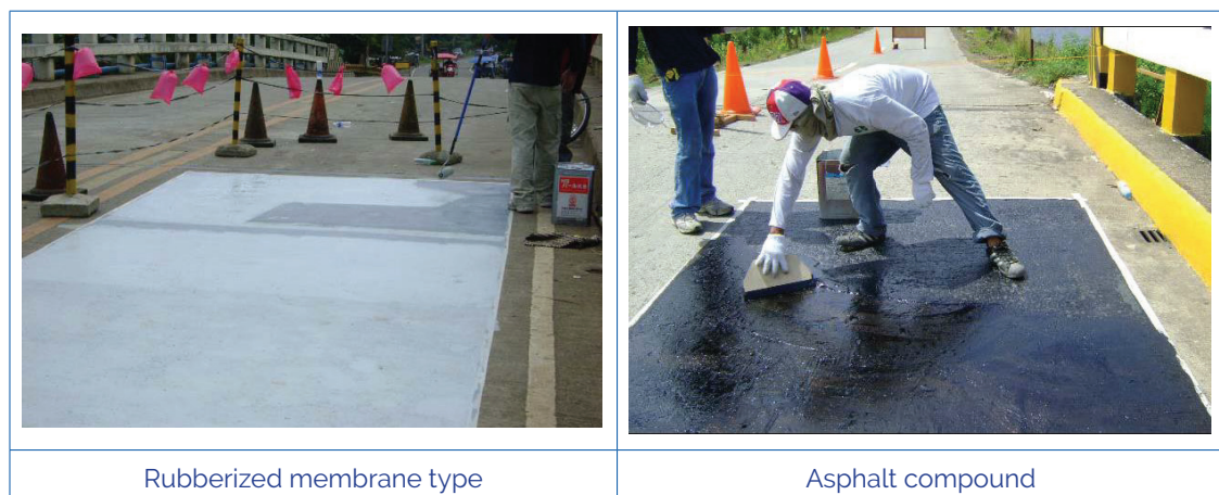
Figure 3.25 Photo illustration of waterproofing
