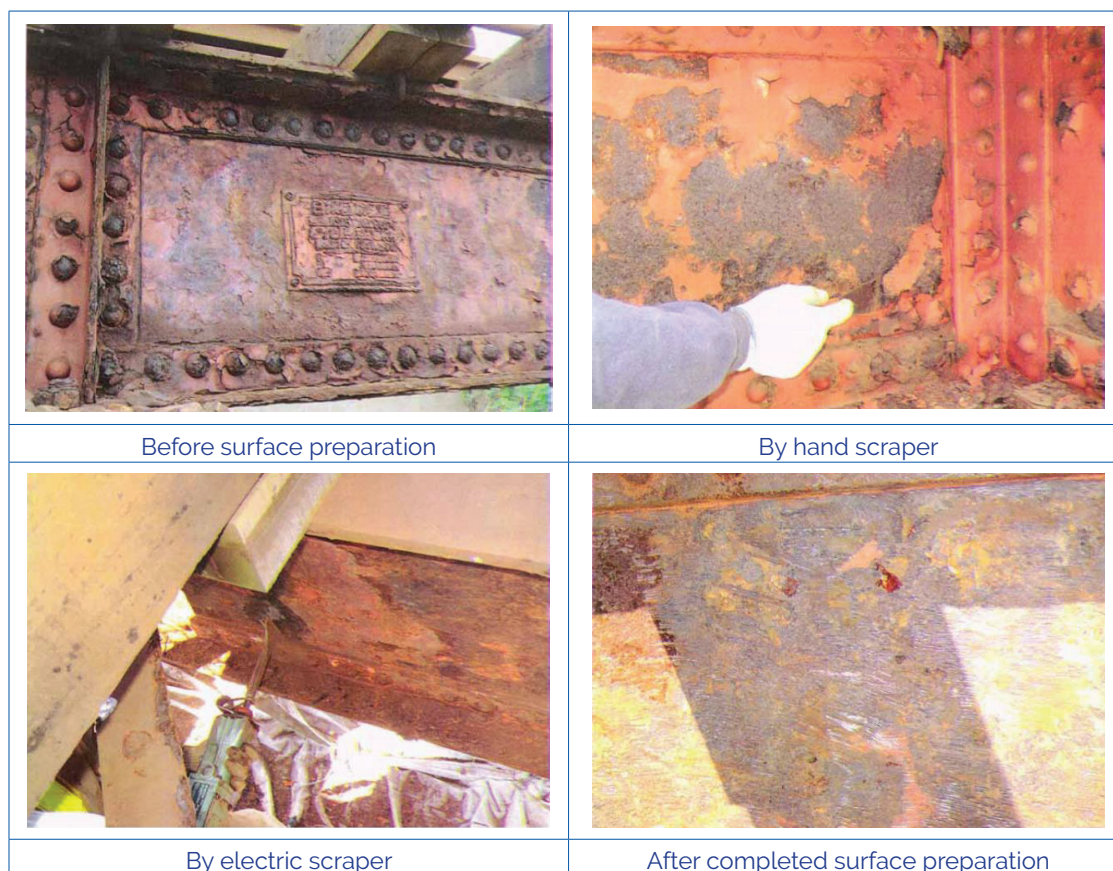
Figure 3.46 Corroded steel surface preparation for painting
