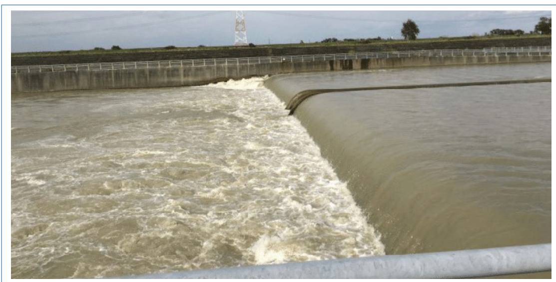
Figure 3.93 Side elevation of a weir
