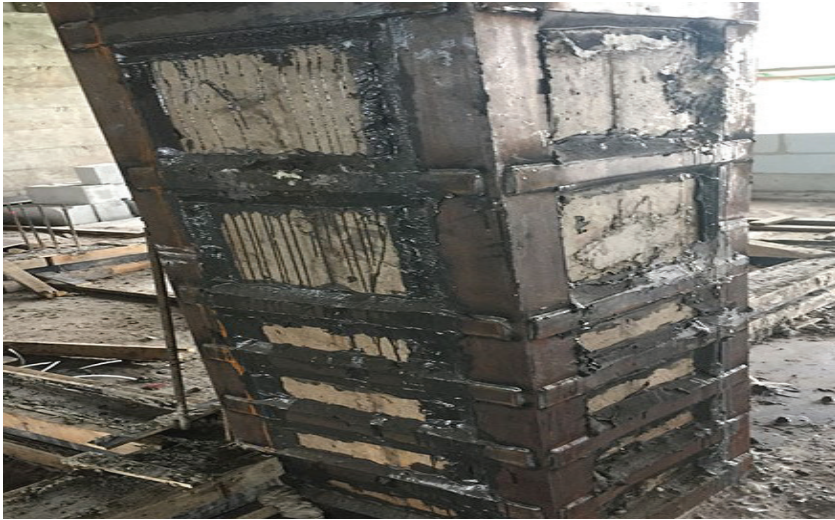
Figure 3.87 Steel jacketing
