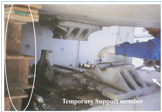
Figure 3.68 Sample of replacement bearing by jacking-up girder
