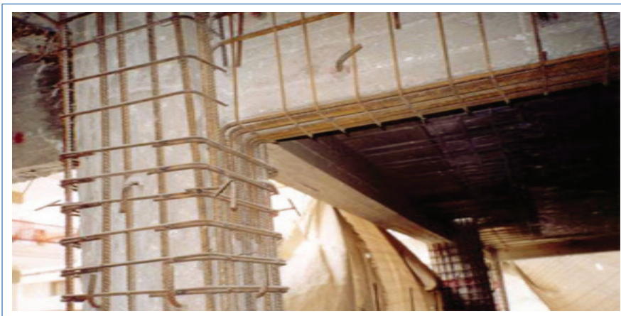
Figure 3.86 Reinforced concrete jacking
