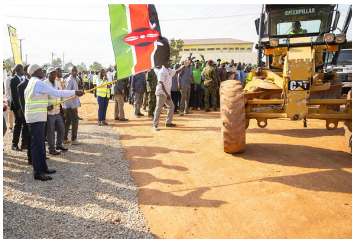
H.E. President William Ruto launches the upgrading to bitumen standards of the 41 km Bukembe-Nzoia Market-Mutomolo Road (C1311/C811)/ Masaek-KDF-Kabariot Roads/County Commissioner's Office-Kijana Wamalwa Referral Hospital Road, Bungoma County on 15 th August, 2026.
